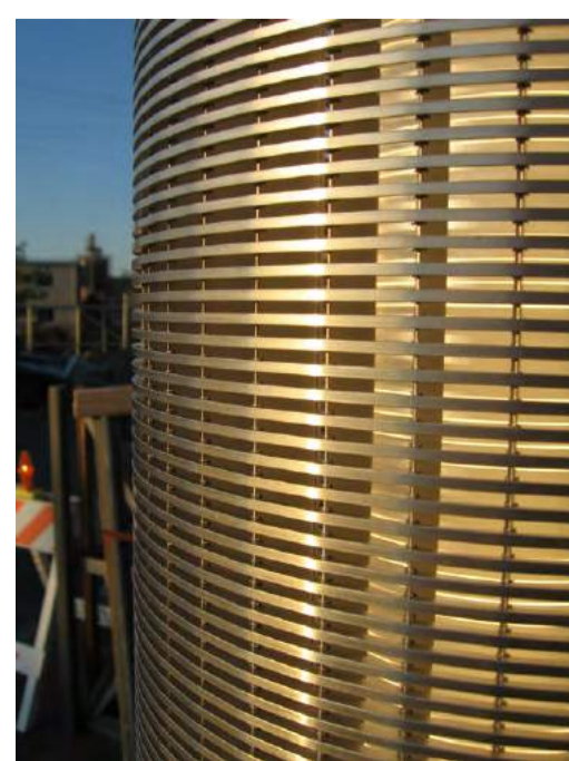
Light emitting mast: stainless steel spiral screen construction
